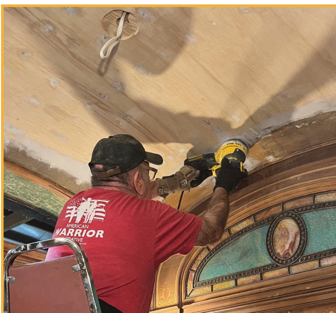
Sanding the epoxy putty along the joints (R) of the upper ceiling and the completed ceiling after all filling and sanding was completed (R).
