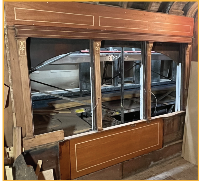
The smoking room outer wall prior to repairs (L) and after the replicated veneer piece were installed (R).
