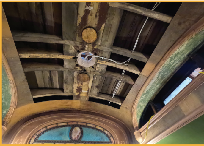
Newly installed electrical wiring routed above the ceiling of the sleeping compartment.
