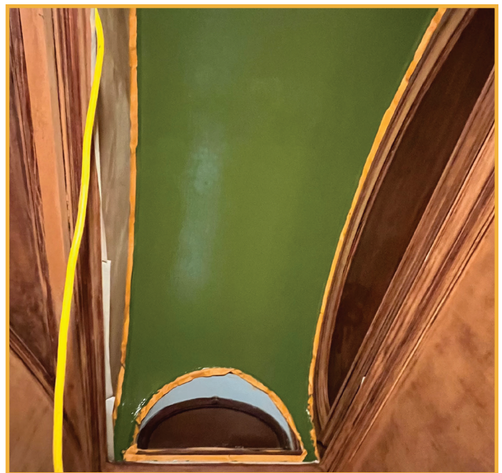
Painting the north east aisle headliner (L) and the freshly painted original ceiling in the Women's Toilet Room.
