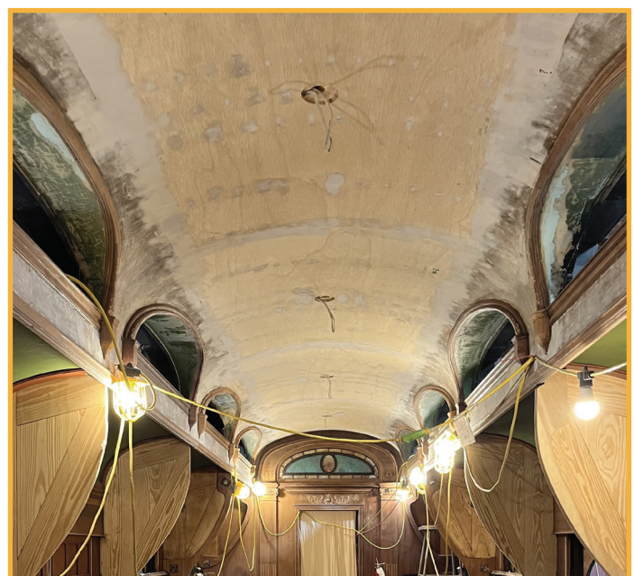
Sanding the epoxy putty along the joints (R) of the upper ceiling and the completed ceiling after all filling and sanding was completed (R).
