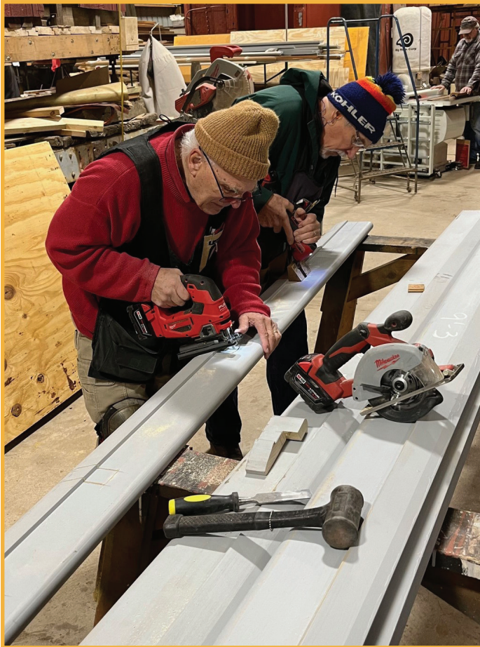
One of the new window sill pieces being trimmed to fit around the car framing (L) and the first new window sill piece in place on the car (R).
