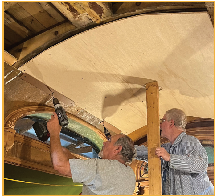
The ceiling area awaiting replacement (L) and volunteers installing the new bending plywood material (R).
